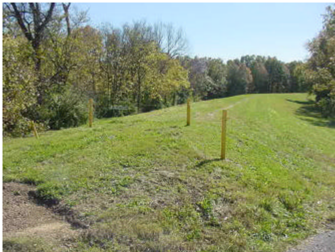
11. Levee at Cairo Road.
