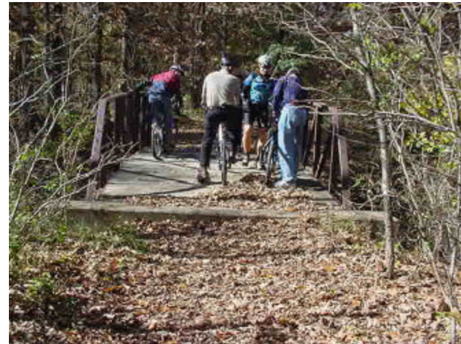
6. Existing bridge between Bluegrass Downs and the levee.
