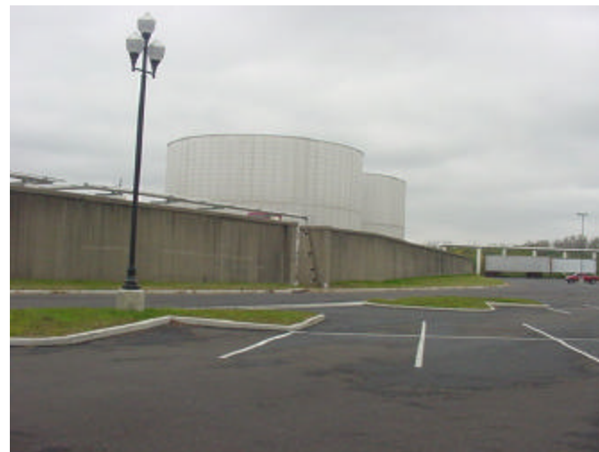
24. Parking and floodwall at the Convention Center.
