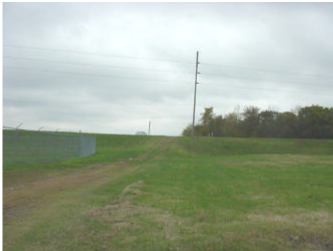
19. Earth ramp to top of levee at Estelle Street and Route 45.
