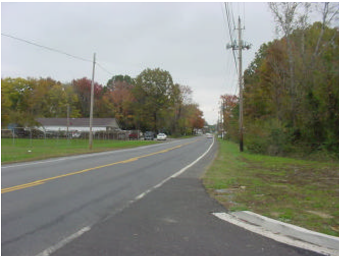
15. View east on Cairo Road at Peck addition.
