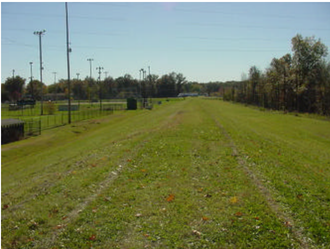
7. Levee at Bob Noble Park where ramps will be located.
