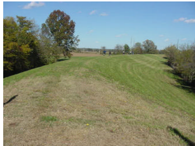
12. Levee between Cairo Road and Route 45.
