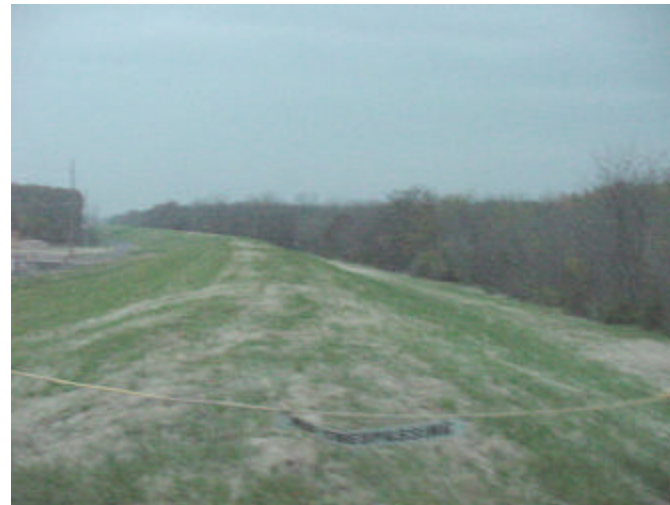
22. Levee between Route 45 and downtown.
