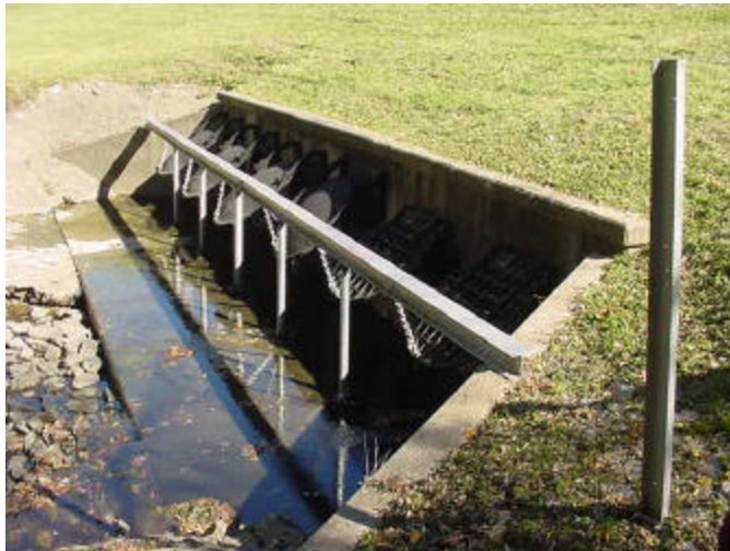
9. Typical outlet structure at pump station.
