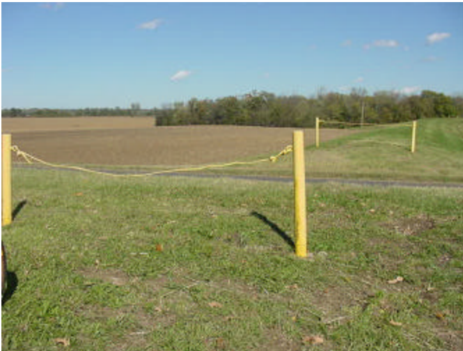
13. Levee at Route 45 crossing.
