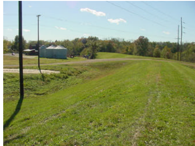
14. Ramp over levee west of Route 45.
